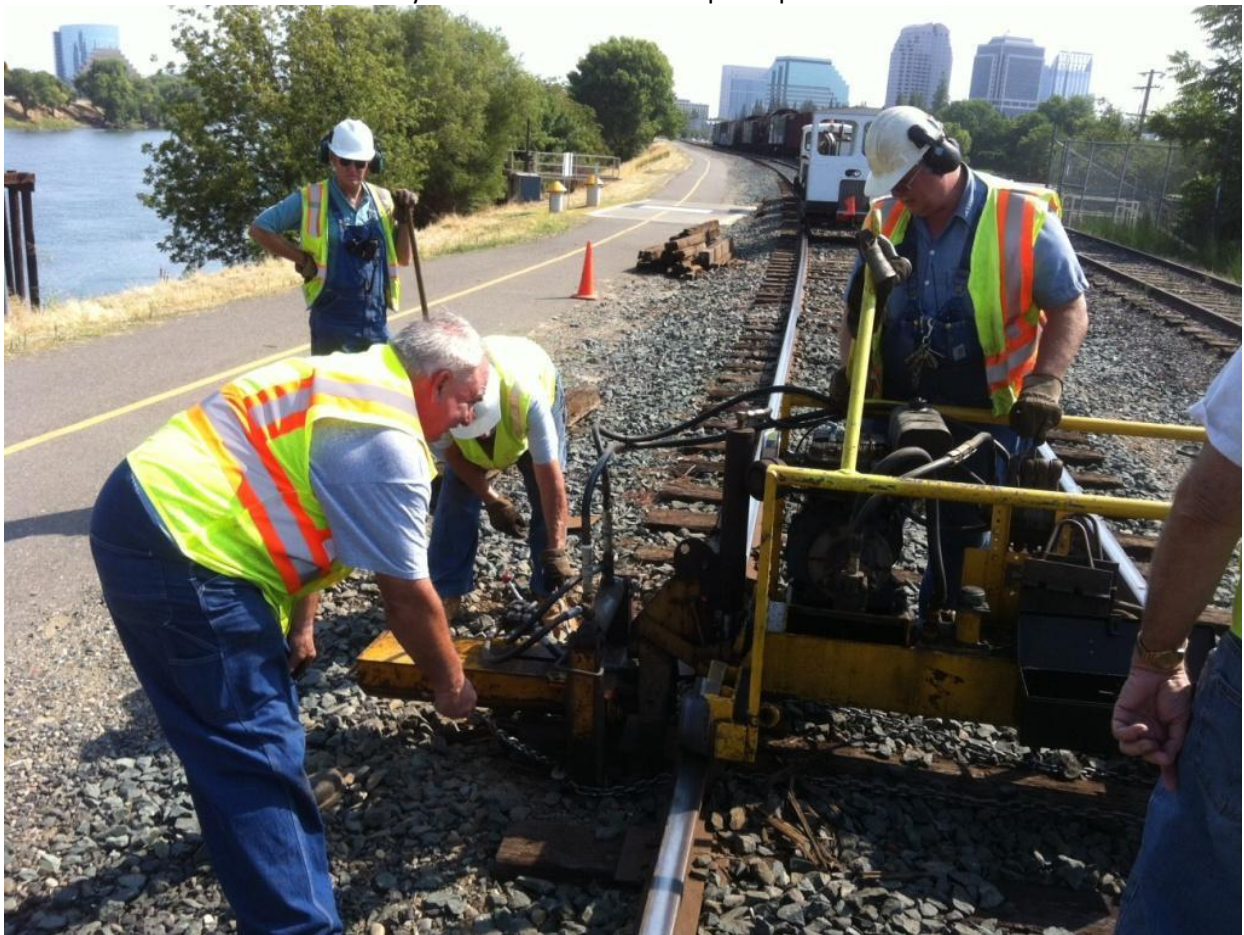
Harry, Clem, Steve, and Chris with the section gang machine removing a splintering tie.
